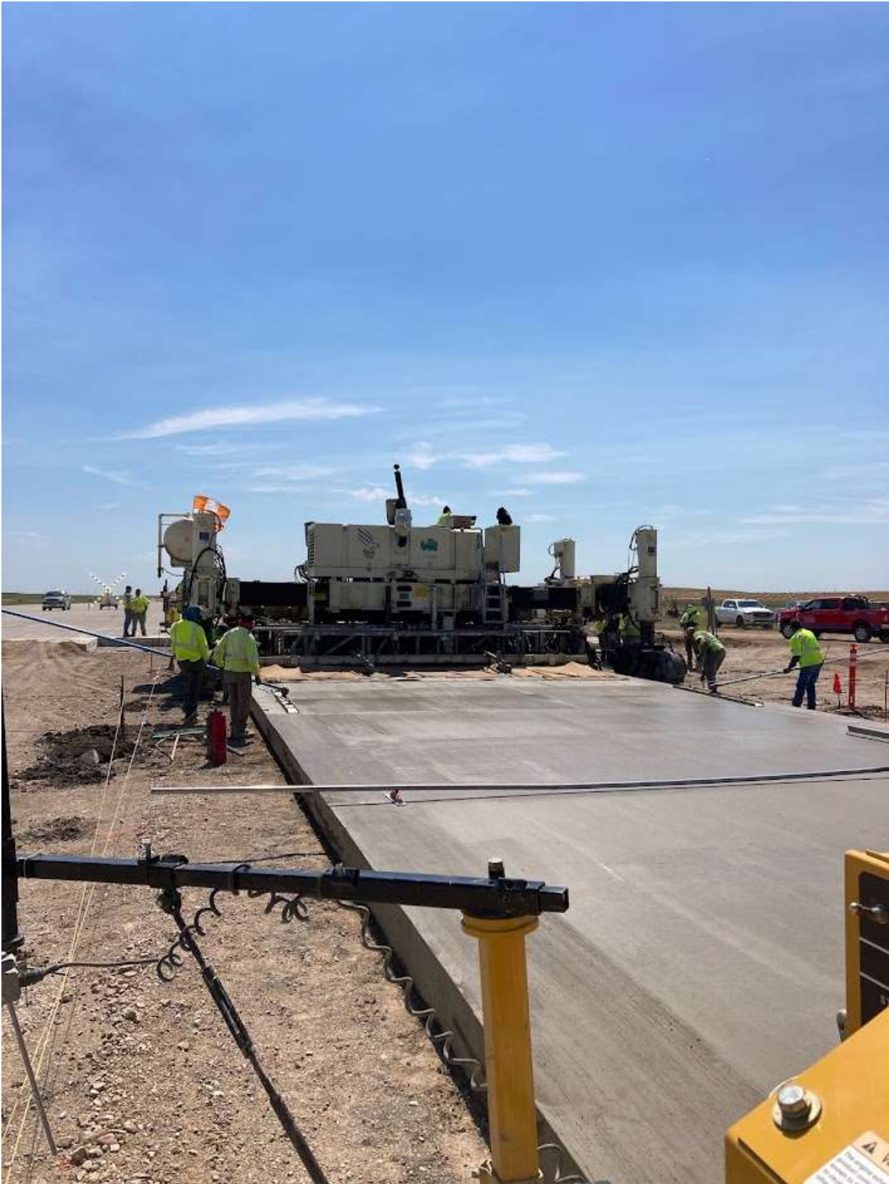
Traveling/Bismarck Concrete – Dickinson Airport Runway
