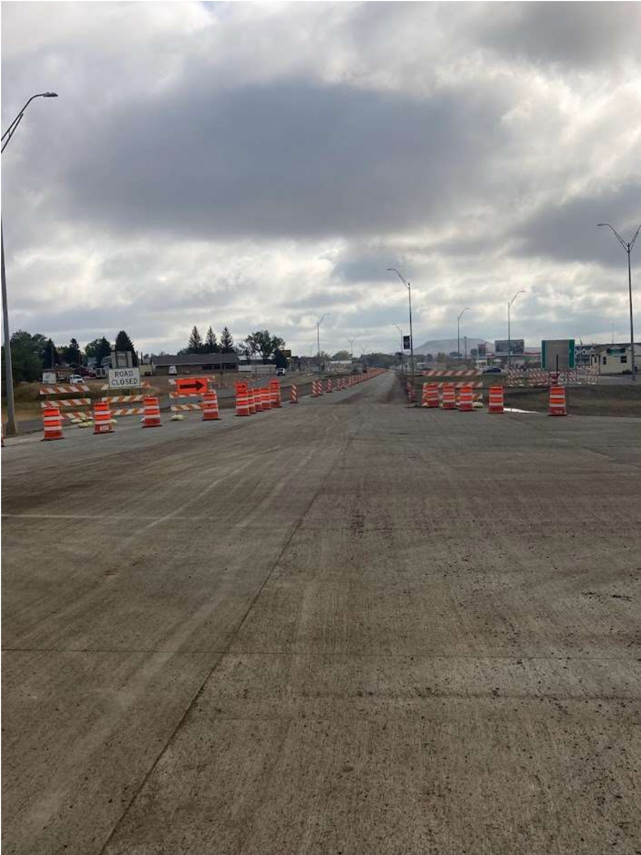
Bowman Project – Traffic Control - Dickinson
