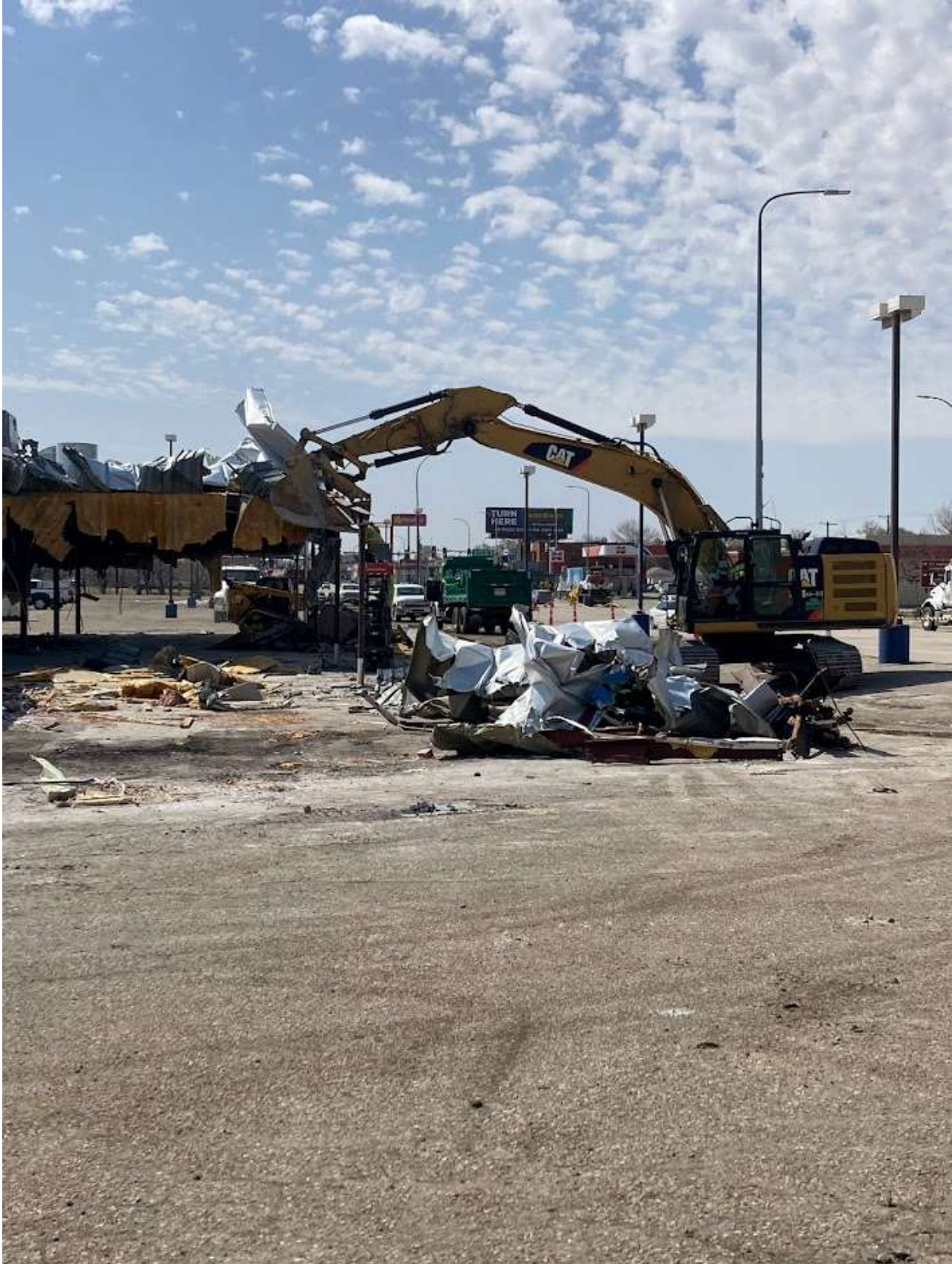
Demolition – Future Hyundai Dealership - Mandan
