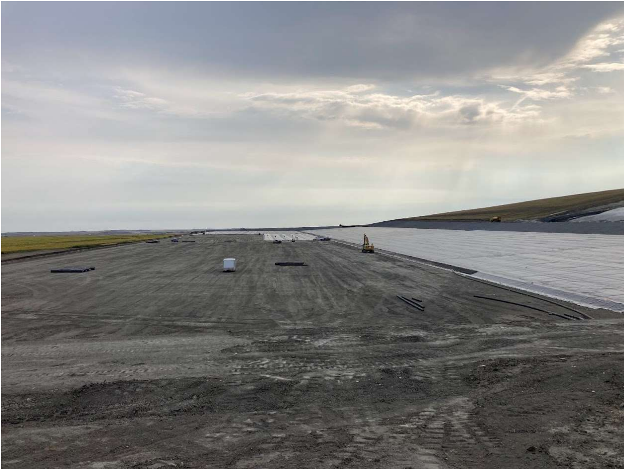
Antelope Valley Station – Cell Construction – Heavy Industrial
