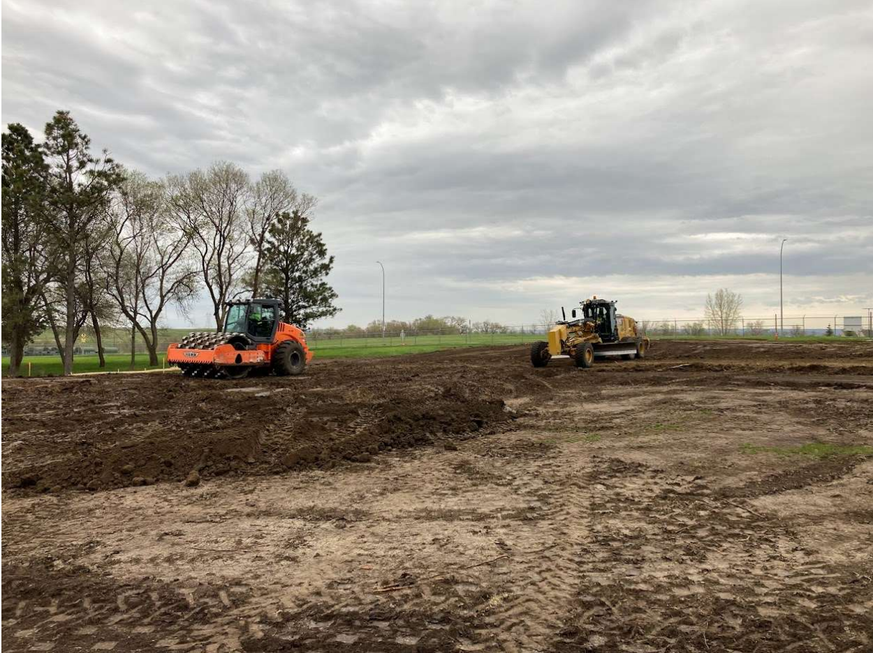
National Guard – RJB Complex – Bismarck
