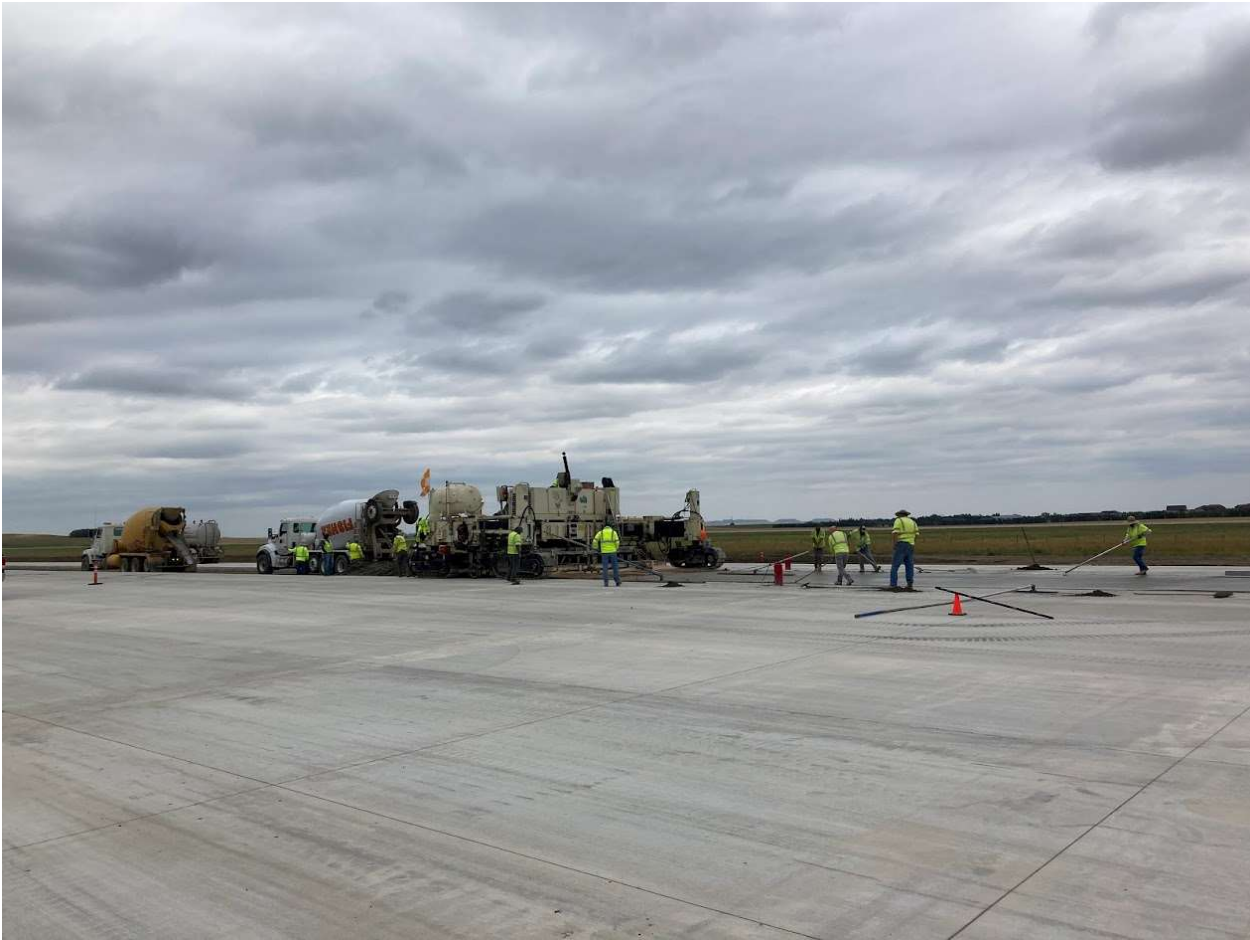
Traveling/Bismarck Concrete – Dickinson Airport Runway
