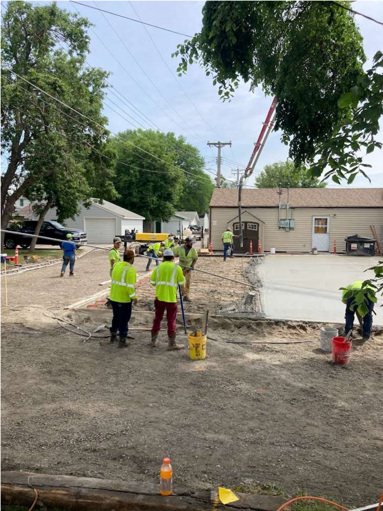
Dilworth – Fargo Concrete
